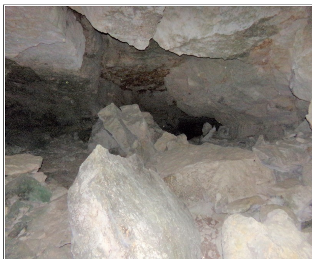
Figure XLI.6: chute de toit massive.
